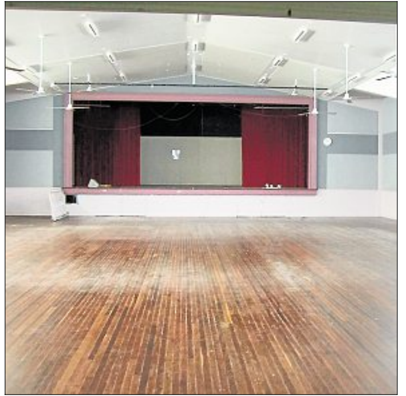
The floor from the old hall has been repolished and installed in the new hall.
